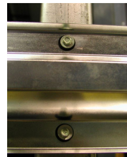
Figure 10.: Connection of the hat section to the C-section
