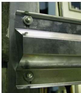
Figure 9.: Hole allowing longitudinal motion of the hat section
