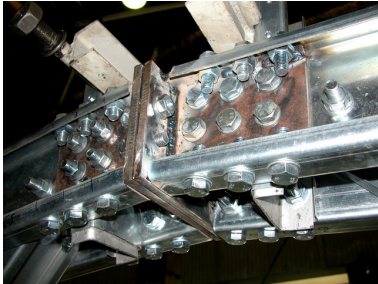
Figure 91.: Ridge joint configuration.
