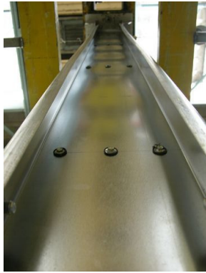
Figure 38.: Local buckling in the web.
