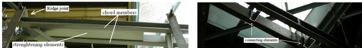
Figure 82.: Strengthening in the upper chord.
